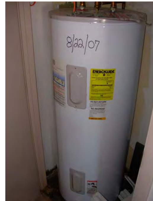
8. DHW tank serving Cmnty. Bldg.
