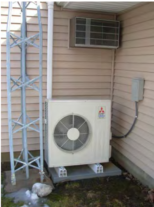
7. Heat pump HVAC system and thru-wall AC serving Community Building Millbrook Village • Capital Needs Assessment • © On-Site Insight
