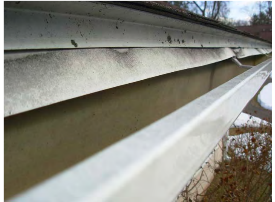
6. Gutters to be adjusted, sectional replacement
